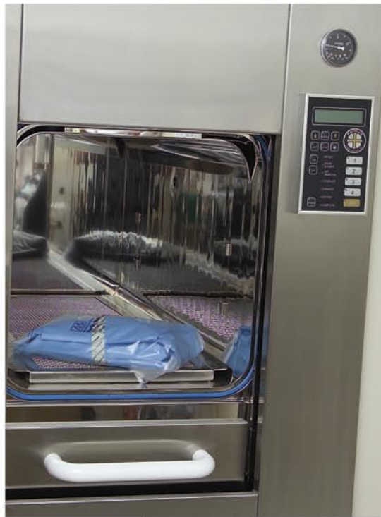
Clockwise from upper left: Before leaving the unit, instruments and other materials must pass through this autoclave, which sterilizes the items. Maintaining ‘negative pressure’ in the biocontainment unit is essential so that contagious organisms do not enter other parts of the hospital. Some items are disinfected after being placed in a bag and being dunked in a tank filled with water and a very mild chemical. Lenaghan holds a timer that is used to verify the amount of time that the items are in the solution.
