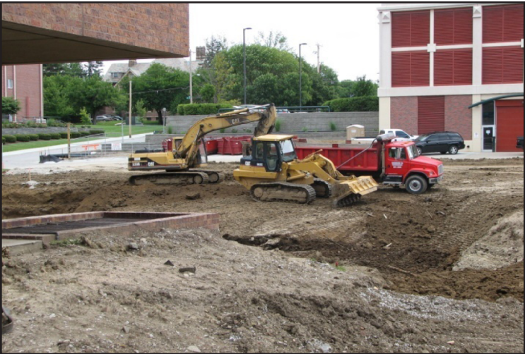
Beginning phase of construction for the College of Nursing Sciences building.
