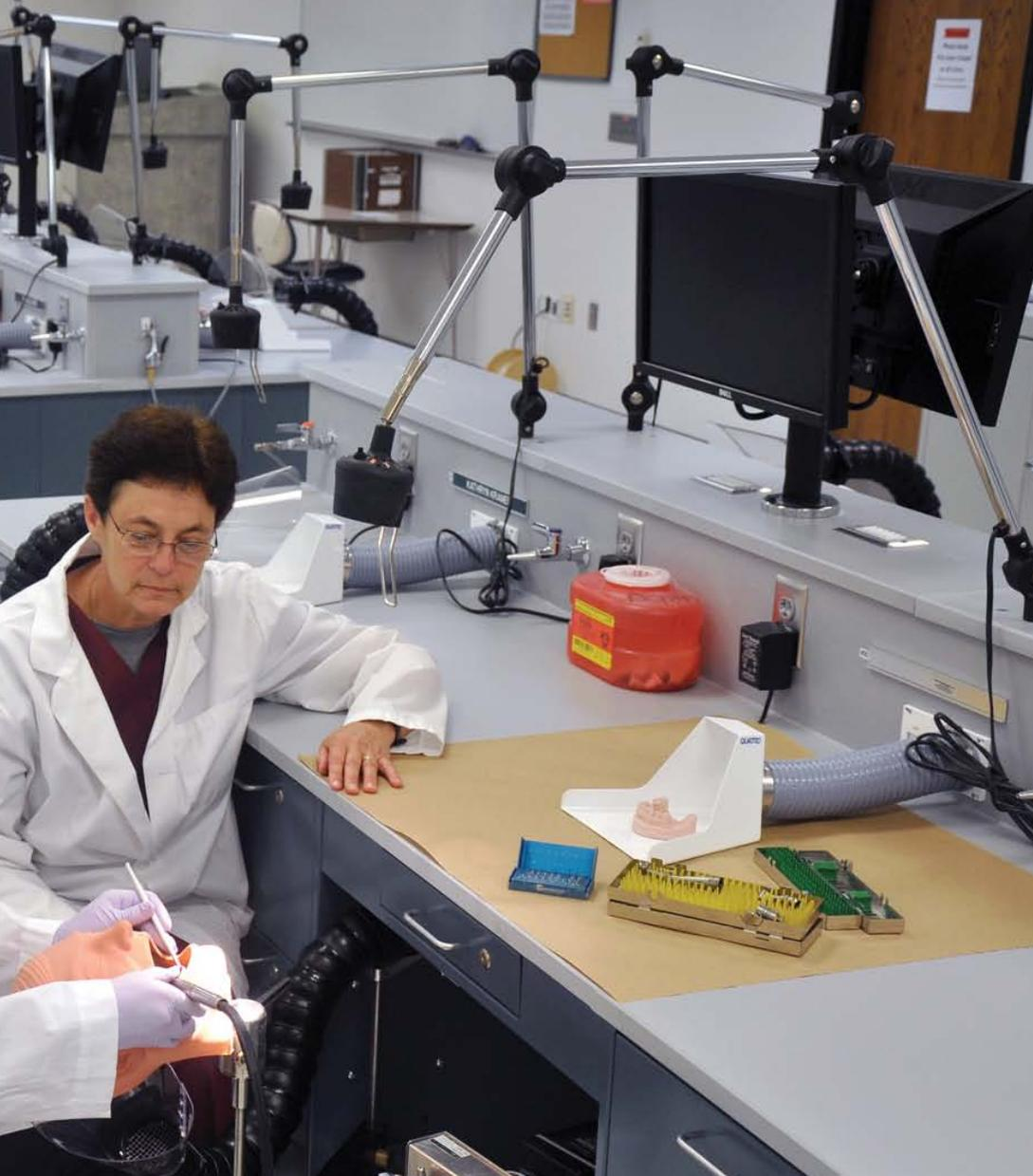
Dental student Katherine Bush works with a manikin while dental aide Bonnie Johnson looks on in one of the two newly remodeled preclinic labs. The new evacuation system is made up of light gray tubing on the counter and black tubing under the counter.
